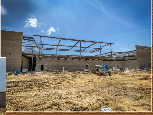
Steel structure and decking on the second floor continue to be installed at the field house.
