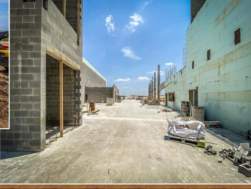
A view of lobby area looking north and south is prepared for CMU block installation. Slab is prepared for concrete pour on the practice gym.
