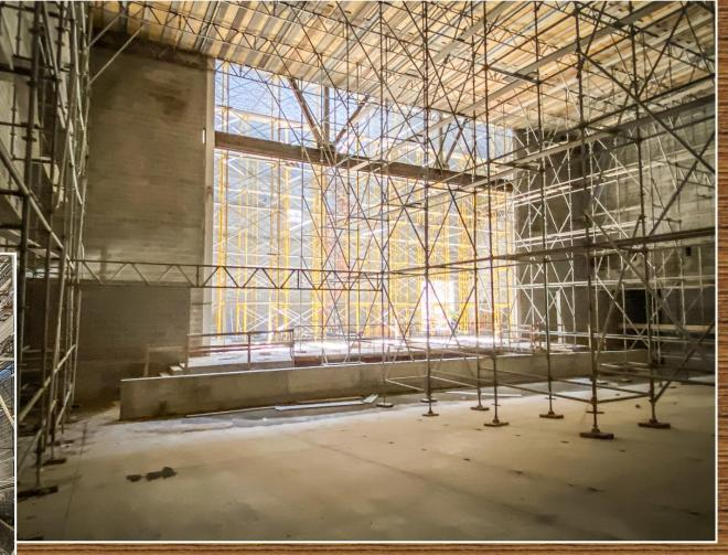
Scaffolding in the PAC interior and fly loft is being prepared to begin work on the above ceiling.
