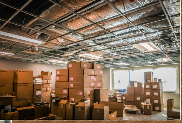
Library ceiling grid has been installed and panels have been delivered.
